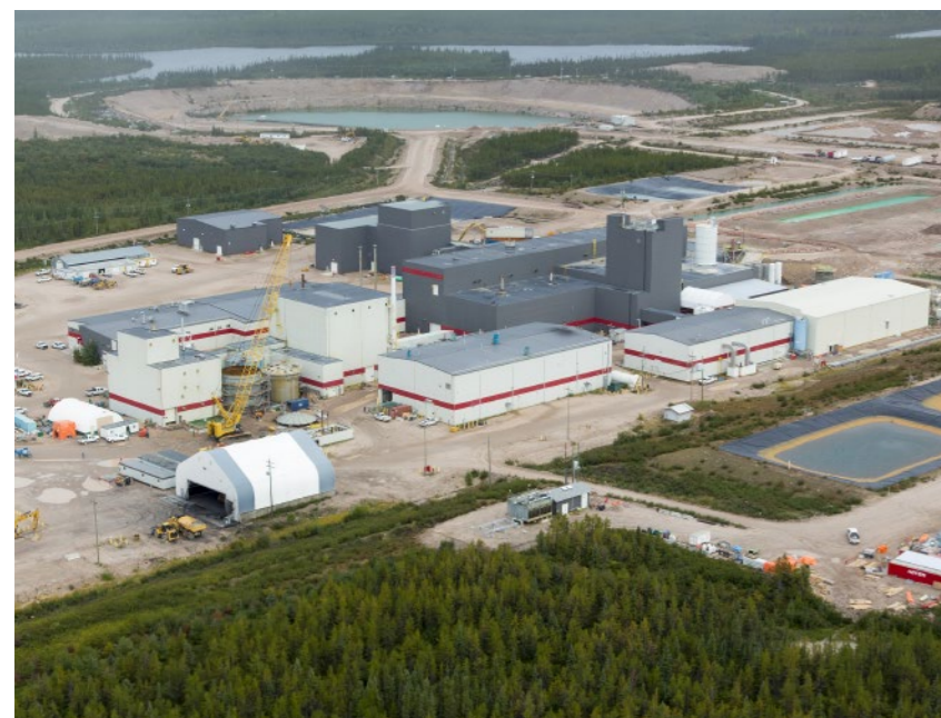
McClean processing plant (Source: Denison Mines)
