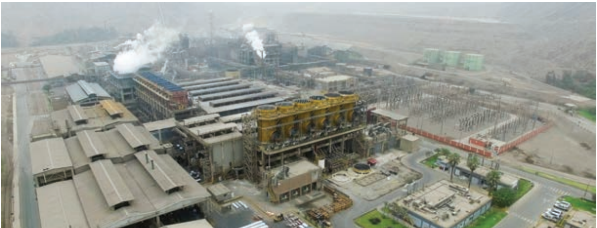
Nexa Resources' Cajamarquilla smelter, 20 km east of Lima, which would treat zinc concentrate from Hilarion. NEXA RESOURCES
