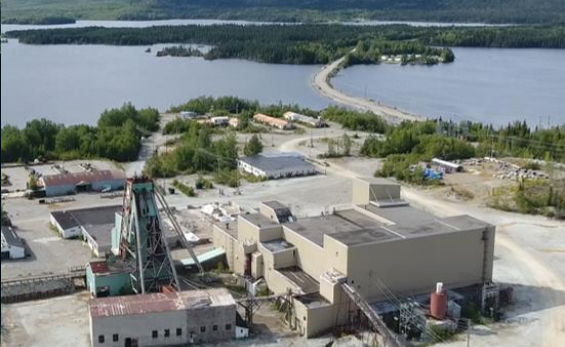
2,700 tpd processing plant
